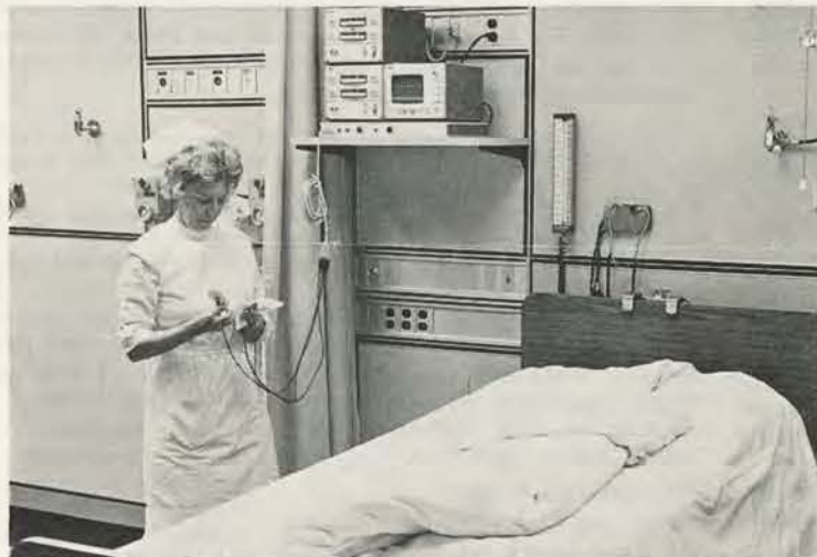
Wall panels contain all equipment for surveillance of individual patients in the newest intensive care units. Each unit has its own power source and suction equipment.
