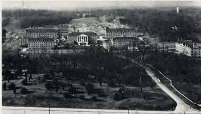
Those were the days when the campus had about 10 permanent buildings, including Top Cottage, which was moved from its site to make way for the CC under construction in the background.
