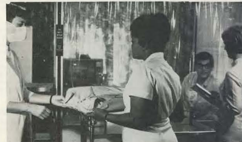
Laminar air flow rooms, developed by the Nursing Department in cooperation with the National Cancer Institute, protect patients unusually susceptible to infection. Ultra clean air flows into the patient's portion of the room, is swept away, and recleaned before flowing back. Patients are observed and treatment is administered through a protective plastic shield. All materials entering patient areas are sterile—even food.
