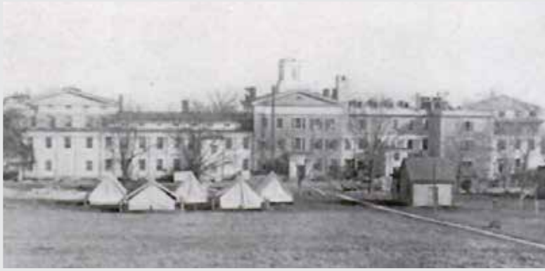
Figure 12. The (west facing) rear of the Marine Hospital, Stapleton, Staten Island New York, where the Hygienic Laboratory was located from 1887–1891. Isolation tents for tuberculosis patients are visible behind the building. Kinyoun instituted this tuberculosis isolation, apparently being among the first to do so, and he urged unsuccessfully that other Marine Hospitals follow suit (31, 32).
