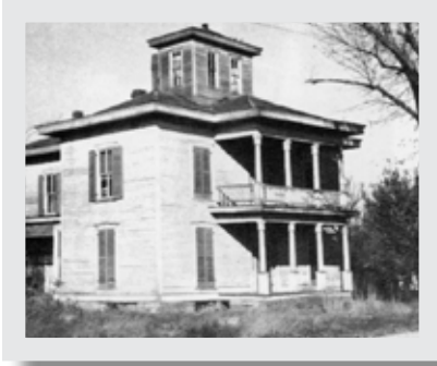
Figure 2. Kinyoun and his family moved to Centre View, Missouri, when Kinyoun was 5 years old (1866). At first they lived in a log cabin but eventually were able to afford a home (12, 18). Kinyoun apparently lived in this house as an older boy or teenager, although the dates of his residence are unknown.
