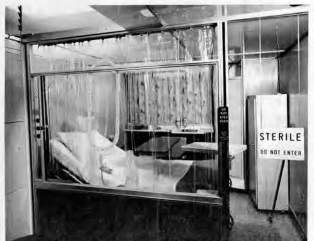
The laminar airflow room, originally designed to assemble space capsules and instruments for use in the NASA program, has a more efficient air filtration system and allows for more patient mobility. (NIH Photo #CC-8)
