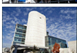
Building 45, the "William H. Natcher Building," is the gateway to the NIH campus. It houses a 1,000-seat auditorium, nine conference rooms, a spacious cafeteria, and underground parking for visitors.
