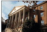
Building 1, the "Shannon Building," serves as NIH headquarters in the heart of the campus in Bethesda, Maryland.
