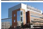
The C.W. Bill Young Center (Building 33) is a new laboratory complex constructed for the National Institute of Allergy and Infectious Diseases (NIAID) to expand its research programs for developing new and improved diagnostics, vaccines, and treatments for emerging diseases caused by infectious agents that may occur naturally or be deliberately released into civilian populations.
