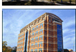
Building 50, "The Louis Stokes Laboratories," provides 250,000 GSF of state-of-the-art laboratory, office and conference facilities for scientists from nine NIH Institutes.
