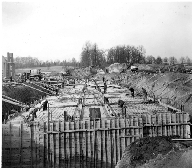
January 1939: Building 6's foundation.
