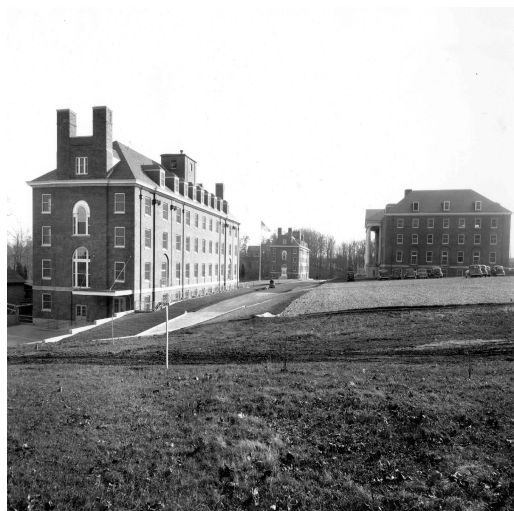
Buildings 1-3 completed Office of NIH History
