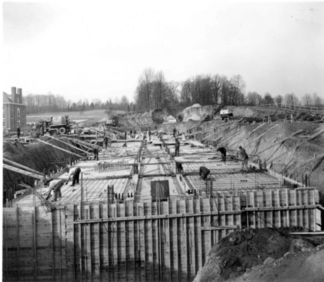
January 1939: Building 6's foundation.
