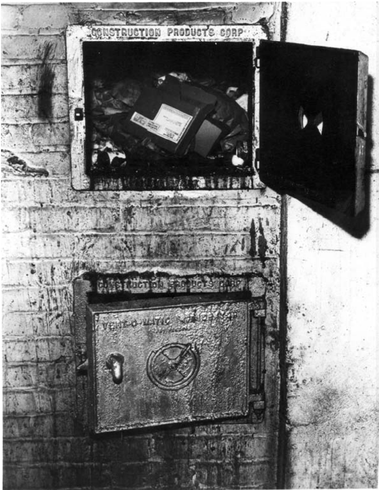
Summer 1946. Incinerators at Kew Gardens. (Office of NIH History files).
